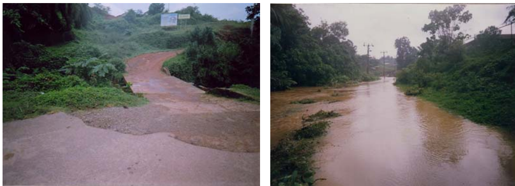
Photo 4: Access Road to the Tea Garden Settlement during Rain and Normal Days
