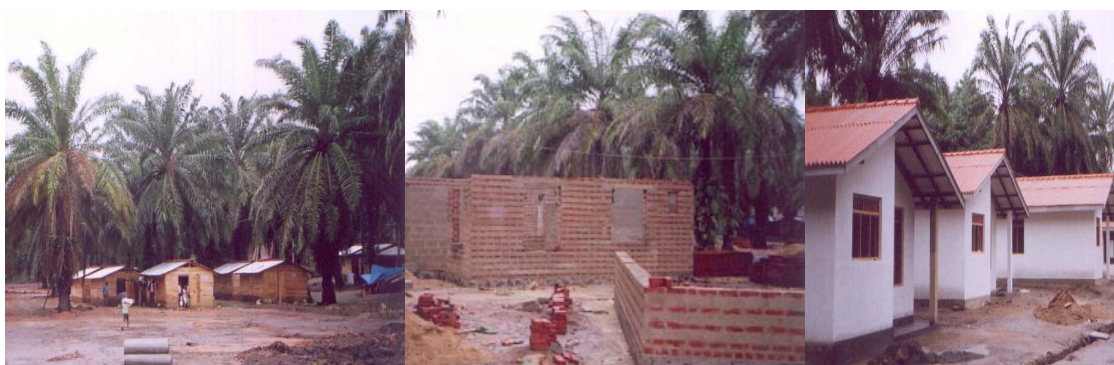
Photo 7: Different stages of housing construction work of Katupolwaththa Settlement
